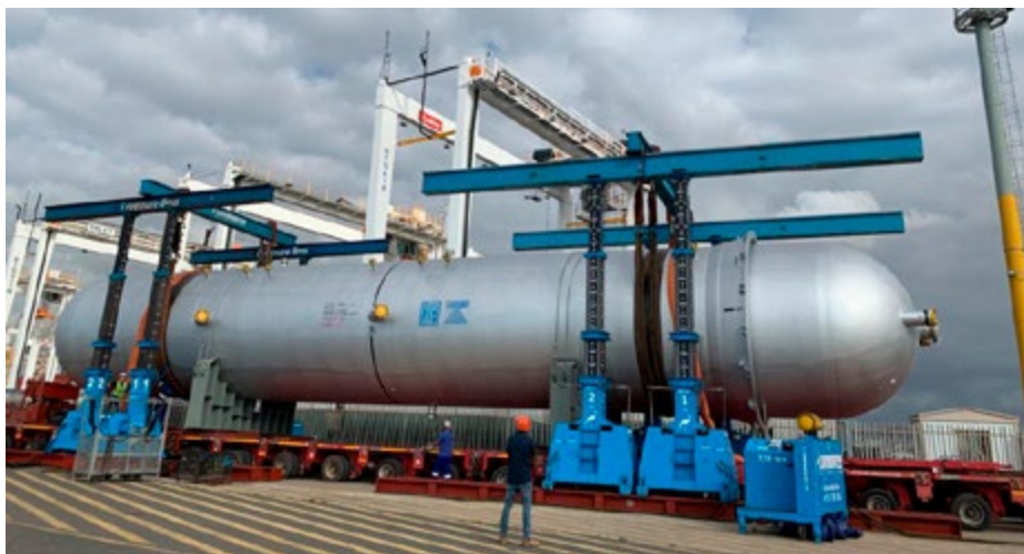
Ton Reactor being jacked up for loading onto trailer.
